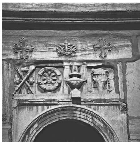
Figure 127 Panagia Gorgoepekoos. Part of a Roman frieze, in secondary use, over the south entrance of the church.
